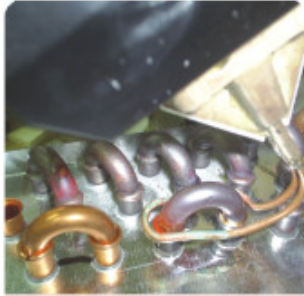
散熱板焊接 Coolers brazing
